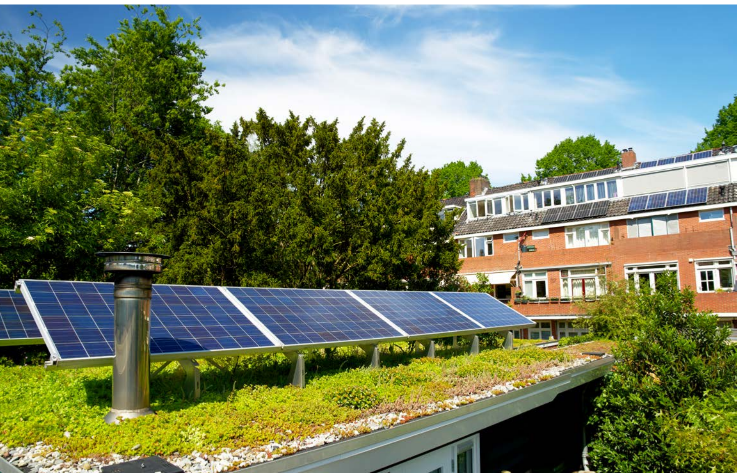
Photo 44: Example image - solar collectors
