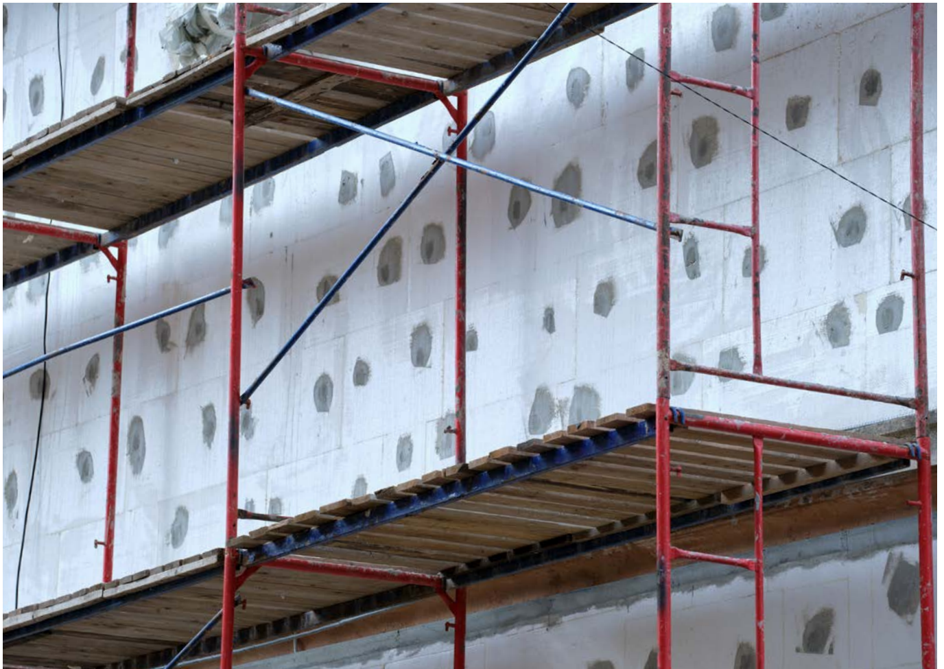
Photo 27: Example image - wall insulation
